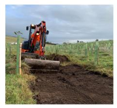
De-Culverting: Due to the area's naturally wet nature, ground mats were used to create a trackway so that water drains away as it works.
